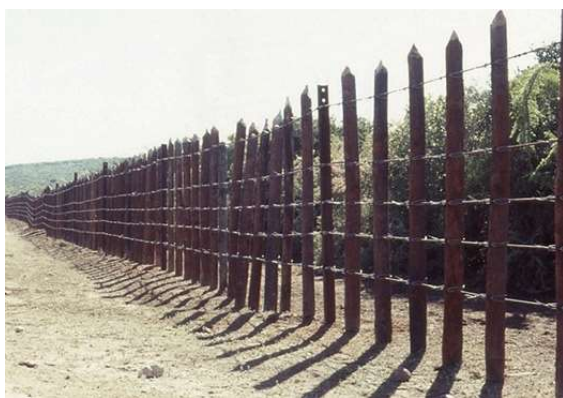
Figure 11 Heavy duty Armstrong fence of Addo NP 1985, RSA Photo: E. Gross. Photo: J. Bothma
